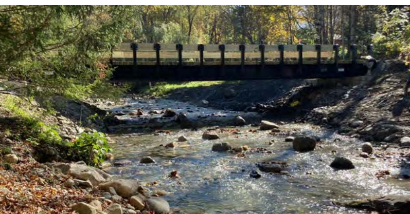
A bridge replacement on the Mettawee River that flows unimpeded.
