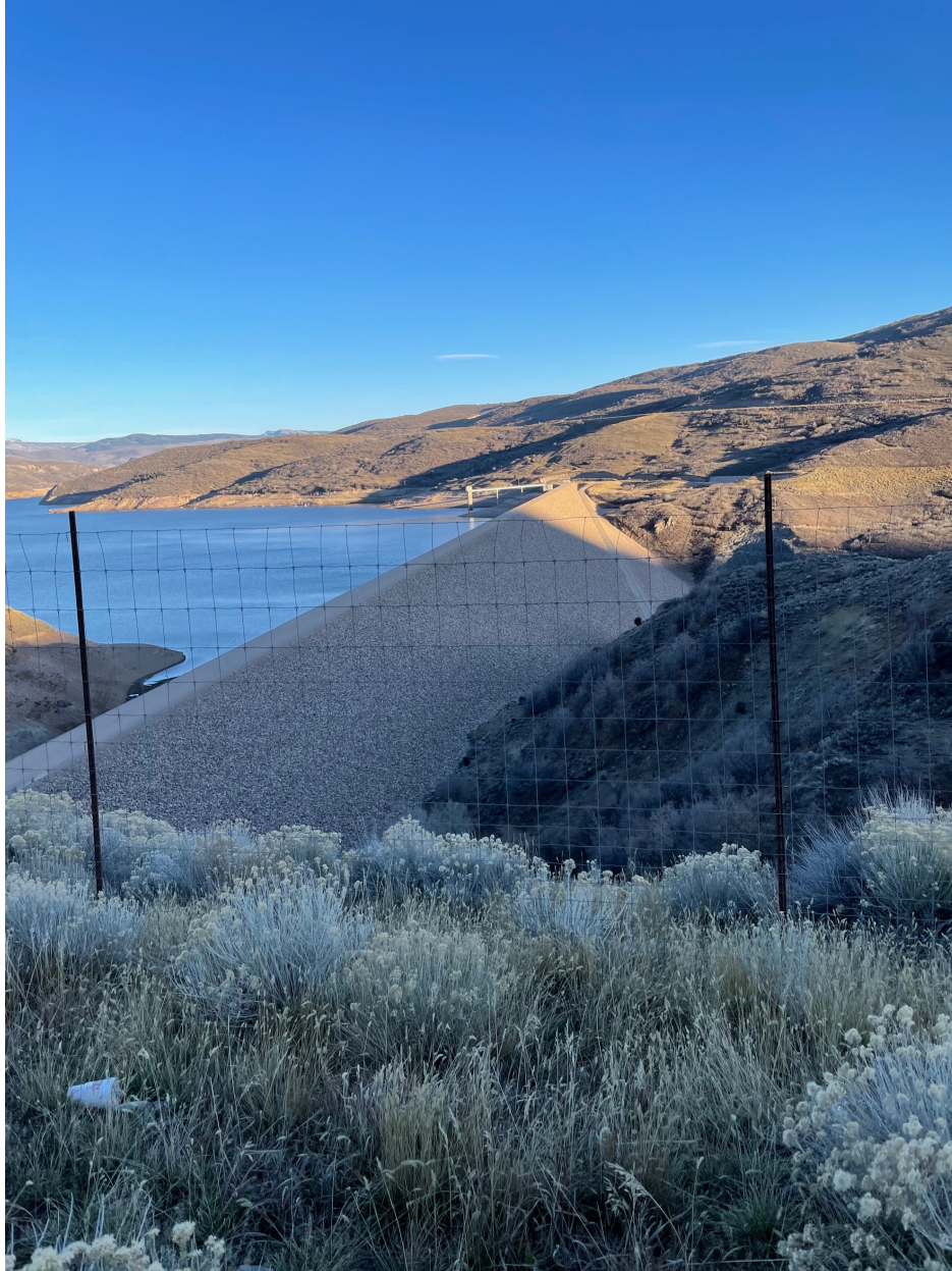
Figure 4. Photo of the Jordanelle dam looking east. In the far distance is the SLOW tower that feeds the dam penstock through one or more of the tower's inlet gates located at different levels in the water.
