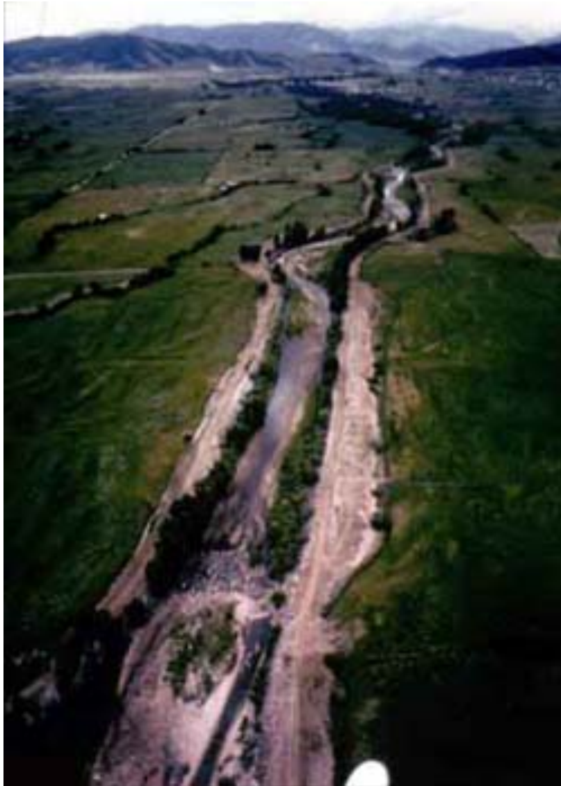
Figure 1513. The pre-Jordanelle channelization of the river. From Provo River Restoration Project .
